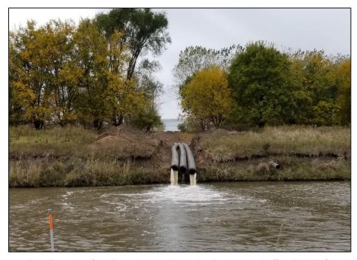
**Photograph 3.** Example of the Return Water Method to Be Used at Buffalo DMMP Site 5, Using Three 20-inch Diameter Pipes Temporarily Placed in an Excavated Gravity-Flow Ditch
